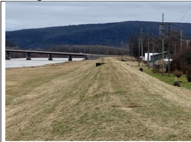
Photograph 6: South Shore Chemung River, Conhocton Street, City of Corning
